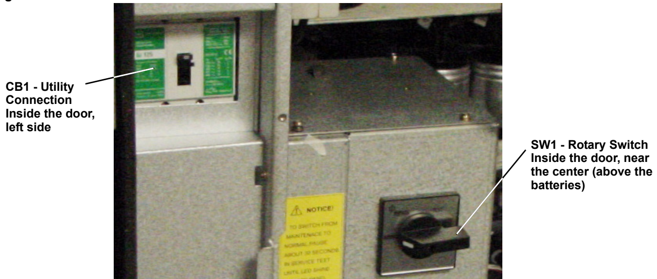
Figure 14 Power switches - 10kVA NX
