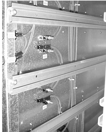
Insert battery drawers in Silcon DP300E
