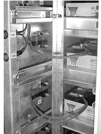
Connect all battery drawers to the terminal on the left side of the column
