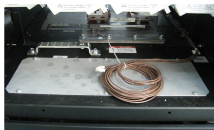
Figure 11-7 - 431B Factory Supplied Shunt Trip Wiring
